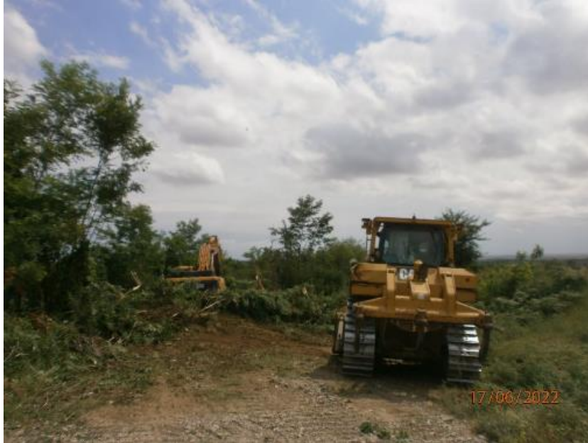
Figure 1 – Contractor’s activities for site Clearance dated 17 th of June 2022
